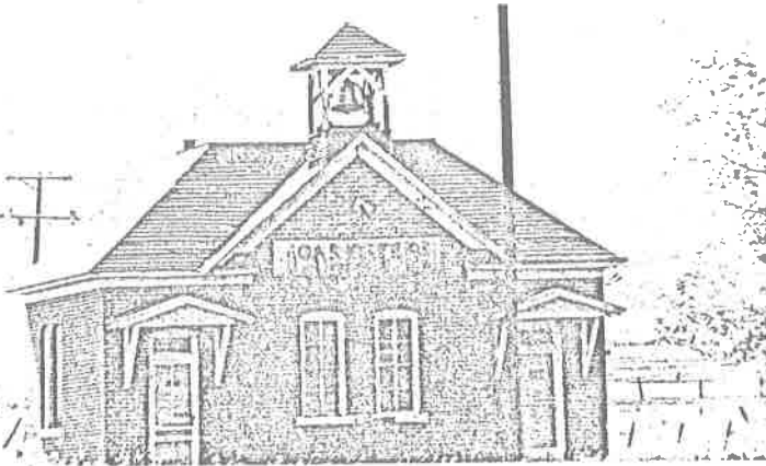
Gas Creek School house 1980, south of Nathrop. Bailey photo.
