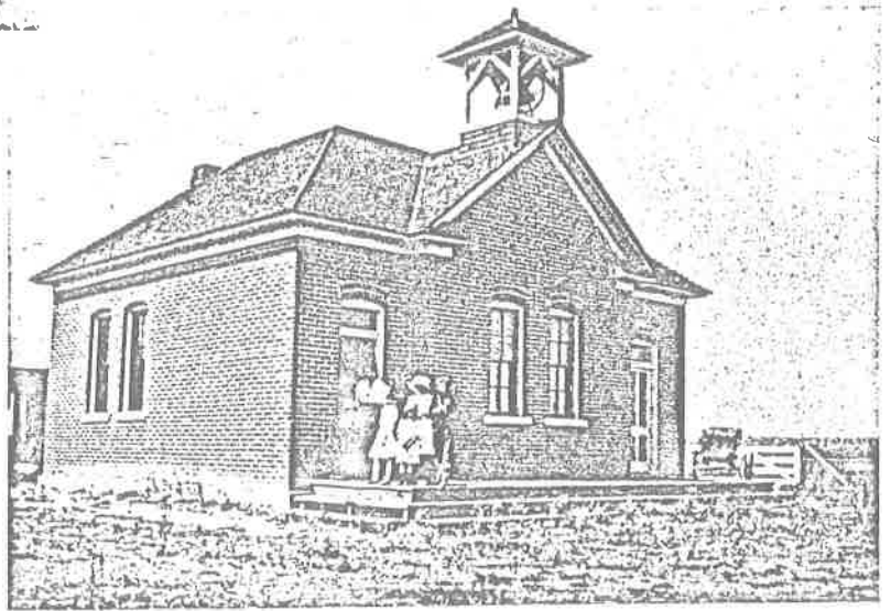
Gas Creek Schoolhouse, late 1980's. Fehling photo.
