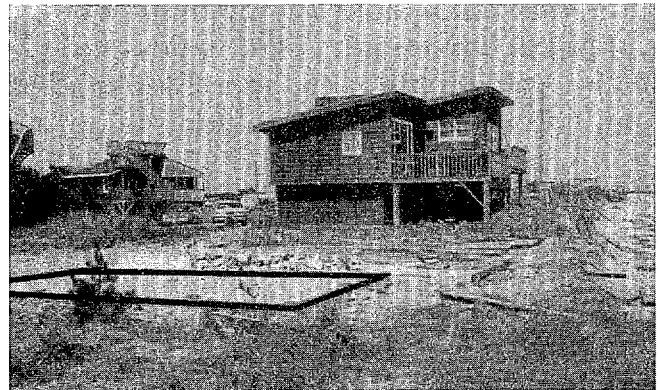
Many jurisdictions require that the old lot be returned to pristine conditions or its natural state. Note the concrete slab and construction materials that must be removed. Some of these lots have remained private property, while others have been utilized for public access to waterfront areas.
