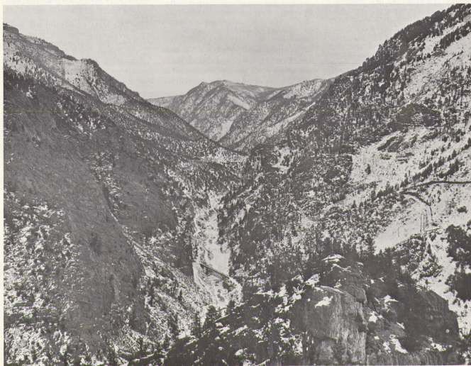
Curecanti Unit — Morrow Point Dam Looking upstream from a high point between Cimarron Creek and the Gunnison River. Morrow Point Dam, a 465-foot high concrete-arch dam, will be located immediately upstream from the railroad bridge across the Gunnison River. Note transmission line access road and Morrow Point-Curecanti 230-kilovolt transmission line structure in right center of photograph.
