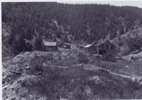
Looking southwest up Long Gulch from the Smuggler tunnel dump, July, 1929. Flood debris in the foreground. Balarat buildings, left to right: Smugger stable, boarding house, superintendent's house, bunk house and tunnel house. Bottom edge of Smuggler shaft dump at extreme right.
