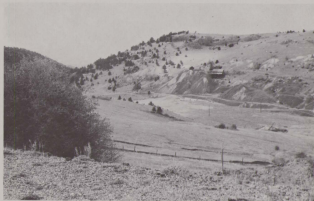
Much of old Aroqua is buried under the tailings pond of the Golden Cycle Mill. The big mine on Beacon Hill is the Gold Dollar.
