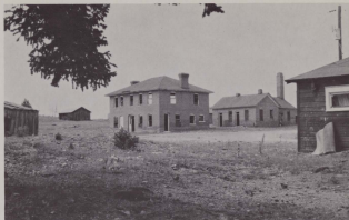
Winfield's big red brick buildings housed offices and laboratories.
