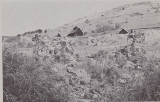
The walls of Anaconda's old jail house frame the few buildings remaining at the Anaconda Mine. (Photo by Dayton Lummis, Jr.)
