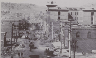
Before the ashes cooled, Cripple Creek began to rebuild. This is how Bennett Avenue looked during the summer of 1896. The big building under construction at the right is the National Hotel. (Denver Public Library Western Collection, Photo by H. S. Poley)
