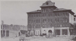
Cripple Creek Builds! The large building under construction is the 150 room National Hotel, the largest and finest hotel ever built in the District. To the left of it, the new Gold Mining Stock Exchange Building is taking shape. (Denver Public Library Western Collection)
