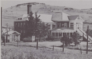
The Cripple Creek Travel Park and Hospitality House, another Macklin development, was once the Teller County Hospital. The old building offers attractive overnight accommodations and the park surround it provides space for campers. (Imperial Hotel Collection)
