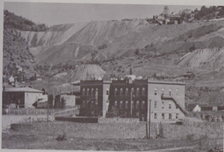
The Ajax Mine on Battle Mountain may soon be a working mine once again. The now deserted Victor High School Building stands in the foreground.
