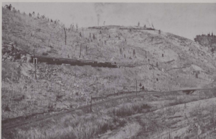
The first rail service into the District was over the narrow gauge Florence and Cripple Creek line. These steep grades were just south of Victor. (Denver Public Library Western Collection)
