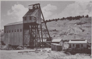
Surface buildings of the rich El Paso Mine, halfway between Cripple Creek and Victor. Deeper than the Empire State Building is high, the El Paso has over thirty-three miles of railed underground diggings.
