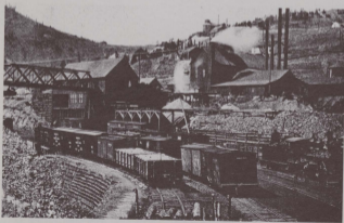
The District yards for the Florence and Cripple Creek were just below the Strong Mine in Victor.
