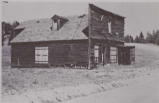
The saloon at Midway. At 10,487 feet, Midway was the highest point in the District to be reached by street cars.
