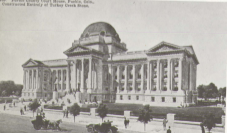
199 - Pueblo County Court House, Pueblo, Colo., constructed entirely of Turkey Creek Stone.
