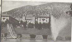
Hotel Colorado and swimming pool, Glenwood Springs. (W-B-T-Co)
