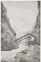
The Hanging Bridge in the Royal Gorge on the Route of the Denver and Rio Grande Railroad, circa 1905. The construction of a rail line through the "Grand Canyon of the Arkansas" was begun in 1878 and completed to Salida in May 1888.
