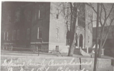
The Gilpin County courthouse, Central City. The county got its name from Colorado's first governor, William Gilpin. The county was established as one of the original counties, formed by the territorial legislature in 1861.
