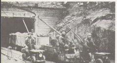
When this photo was taken at the Newhouse mine tunnel at Idaho Springs, the company had installed electric equipment for moving men and ore.
