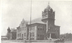
Huerfano County courthouse, Walsenburg. The county gets its name from the Huerfano River. It was one of the 17 original counties formed in 1861.
