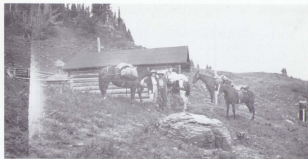
The Flat Tops Deep Lake Ranger Station.
