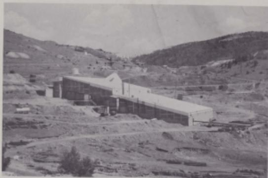
In 1951, the \$1,309,609 Carlton Mill opened between Cripple Creek and Victor with a capacity of 1,000 tons of ore per day. It operated until 1982. Owned by the Golden Cycle Corporation of Colorado Springs, it is still considered the world's largest custom gold mill and one of the best equipped. (Photo by Maxine Adams)
