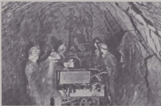
The Carlson Drainage Tunnel, completed in 1941, lowered the water level in the big mines so they could be worked to greater depths. The bore was over 32,000 feet long and cost \$1,046,000. The water it drained off, at the rate of up to 125,000 gallons per minute, went into the Arkansas River and was used to irrigate farms in Eastern Colorado. (Denver Public Library Western Collection)
